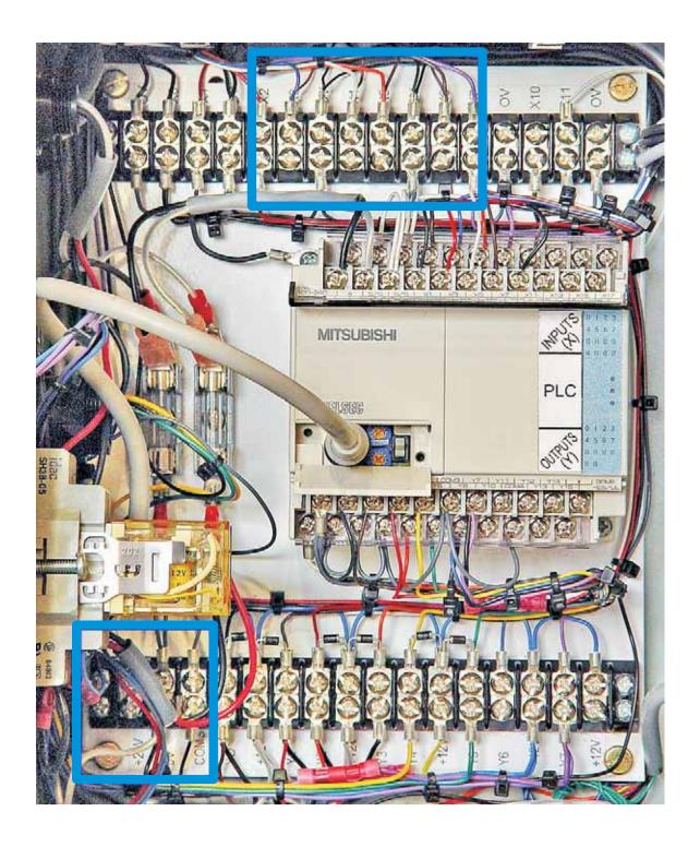
The blue rectangles in the photo above indicates the areas in the earliest (PLC-20) cabinet that re-wiring must be done.
