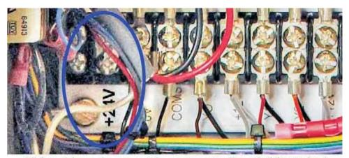
All four blue wires must be connected to +24V terminal
